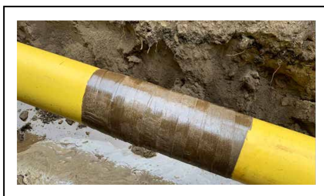
Figure 1. Typical coated gas pipeline showing Yellow Jacket coating and field joint insulation
